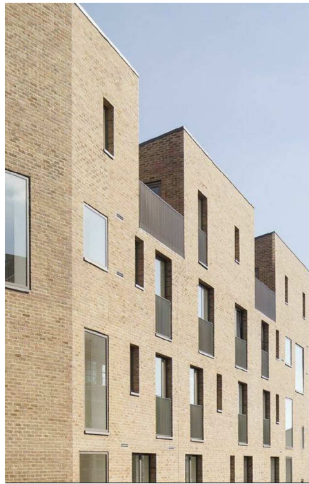
1 PROPOSED LIGHT BRICKWORK FACADE
