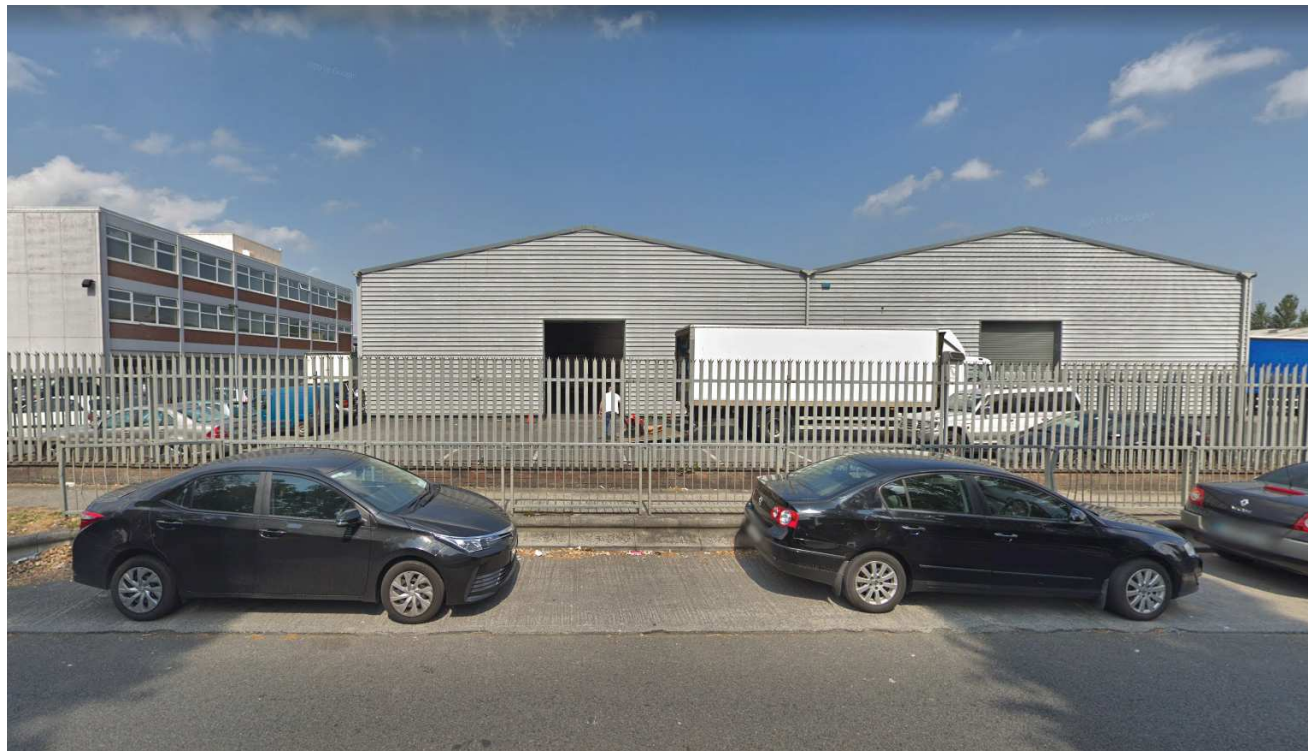
2. View of the SW Boundary of Block B from the Cookstown Road.
