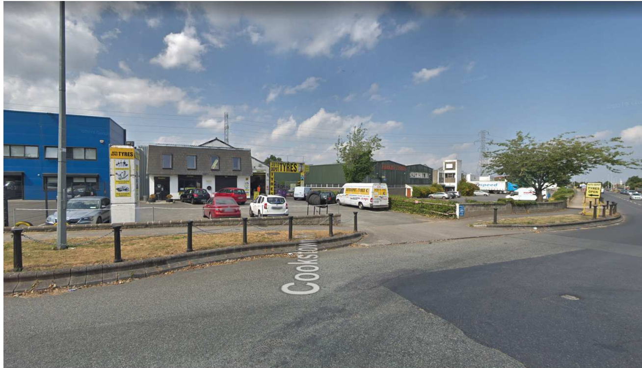
1. View of Block A from the Cookstown Road / First Avenue roundabout.
