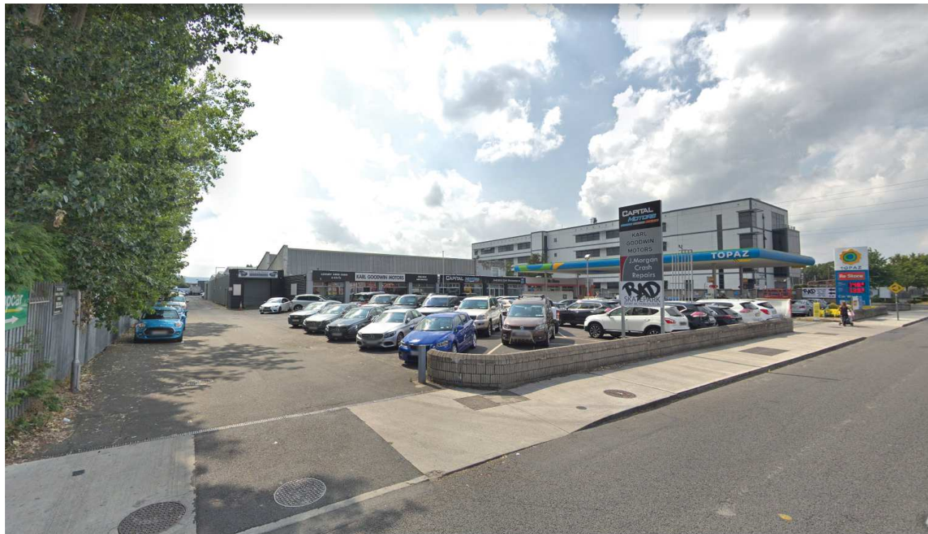
2. View of Block D from the Old Belgard Road.
